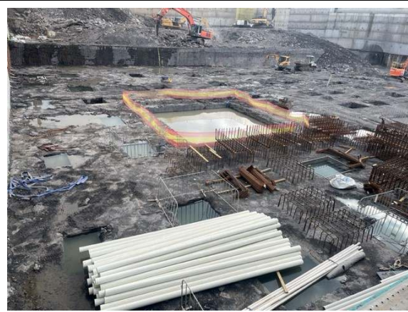
Photos 13 & 14: Sediment basin capturing site runoff for discharge offsite. Spoil load-out continuing on the high-side of the site.
