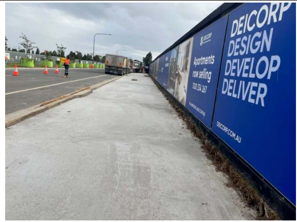
Photos 5-8: Conferta Avenue – lane closure and traffic control in place. Previous nature strip in use for trucks to receive spoil and deliver concrete and materials
