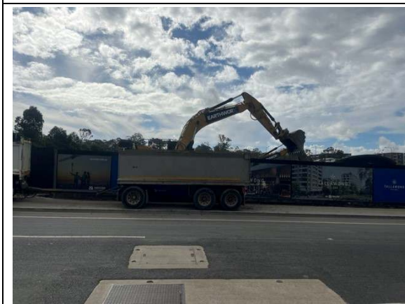
Photos 3 & 4: Spoil load-out and concrete pours over the hoarding on Conferta Avenue
