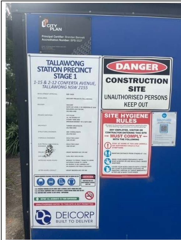
Photo 1: Compliant site signage at entry
