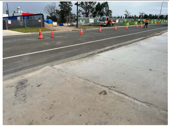
Photos 5-8: Conferta Avenue – lane closure and traffic control in place. Previous nature strip in use for trucks to receive spoil and deliver concrete and materials
