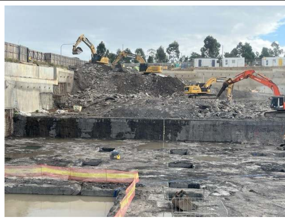
Photos 13 & 14: Sediment basin capturing site runoff for discharge offsite. Spoil load-out continuing on the high-side of the site.
